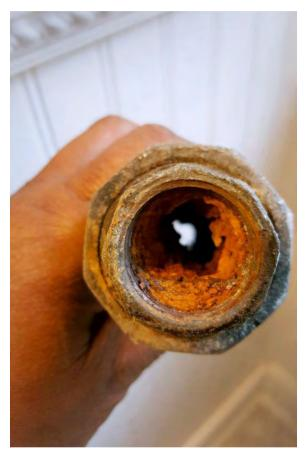
State Rep. LaTonya Johnson, D-Milwaukee, holds corroded galvanized plumbing that was removed from her Milwaukee house. Galvanized pipes, likely to be in older homes, can accumulate lead from service lines, such as the one supplying Johnson's home.
