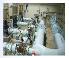
**Wastewater Treatment Plant -** This locally-owned public power utility made several upgrades at their plant and used RFP funding to install a high-efficiency blower with a variable frequency drive, as well as additional aeration piping and blower control system upgrades. These energy efficient upgrades made it possible to reduce expenses, better serve ratepayers, and run the wastewater treatment plant more effectively.
