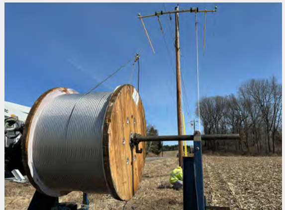
Pictured: Lineworkers running new wire on Halverson Road.
