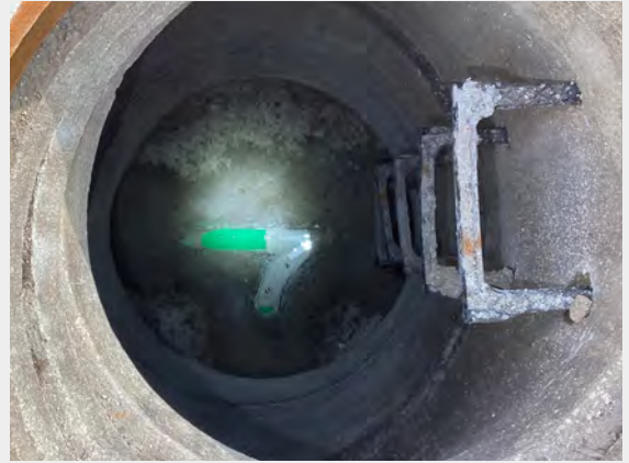
Pictured: The inside of one of the sewer manholes on N Page Street that was repaired this month. Repair was required because the previous state of the manhole caused debris to get caught, requiring monthly cleaning by Wastewater staff. Photo courtesy of Kevin Hudson.
