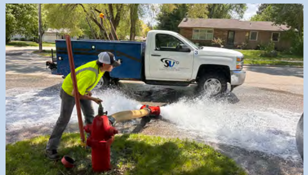
Pictured: Water Operator Dustin K. flushing hydrants as part of our annual hydrant flushing effort.
