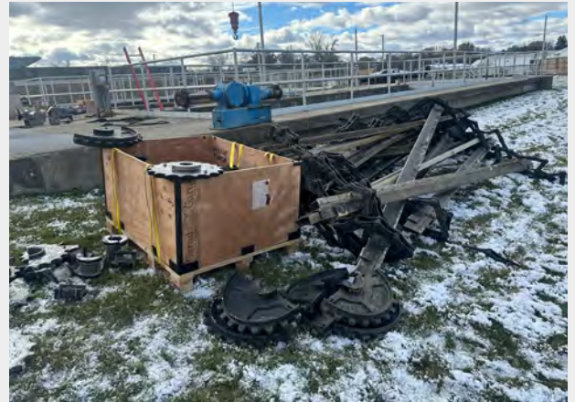
Pictured: Equipment at the bottom of one of the primary clarifiers at the Wastewater Treatment Plant were replaced in November.
